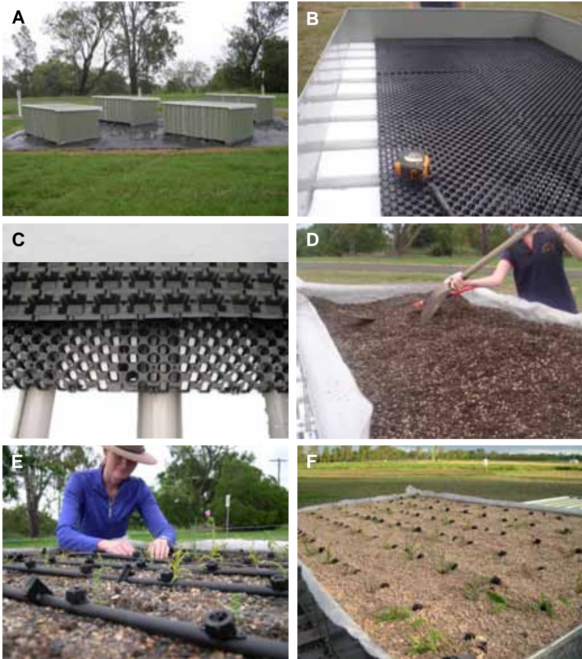
Figure 2. Stages involved in the extensive green roof installation
