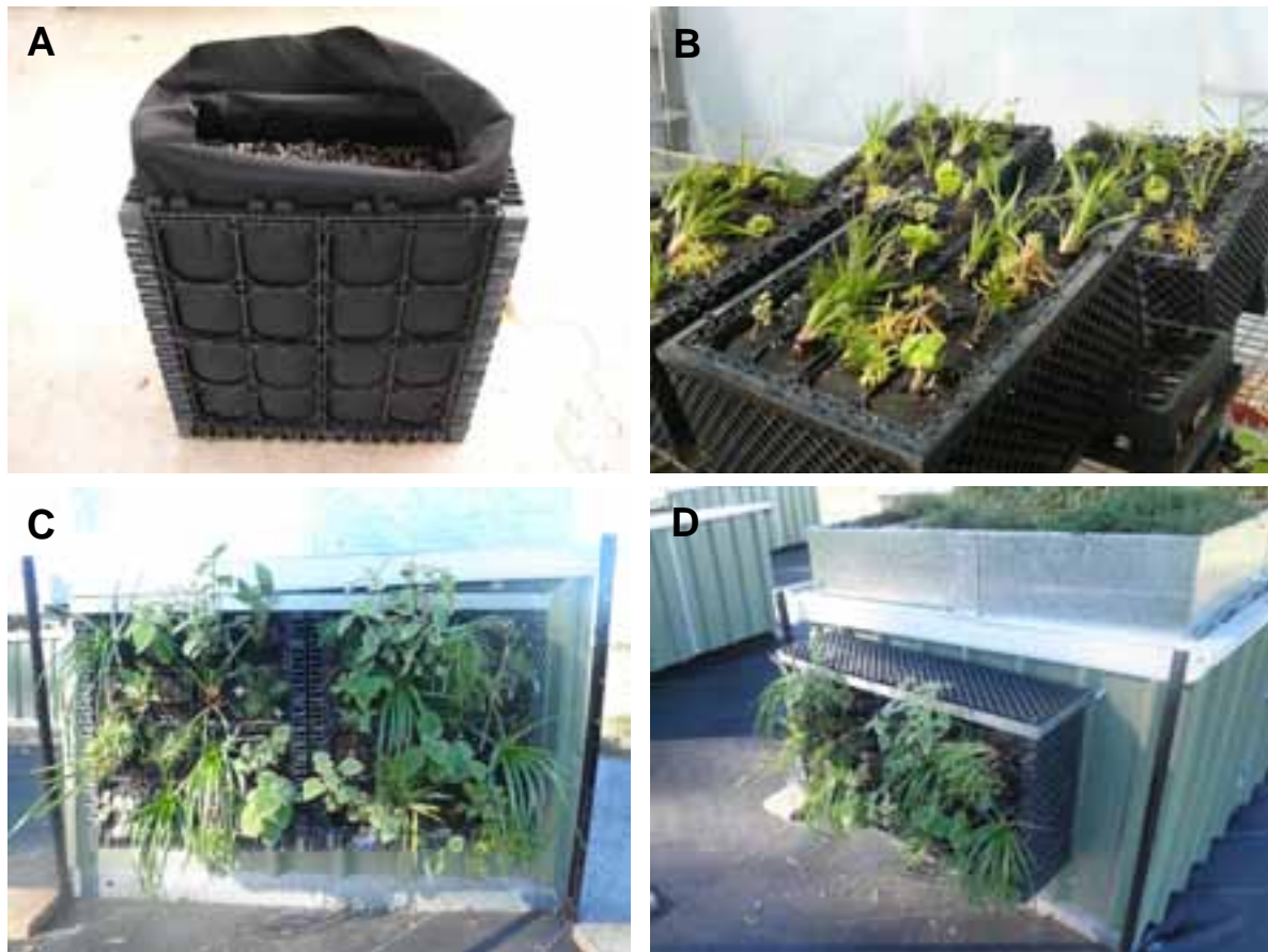
Figure 10. Stages involved in the green wall installation
